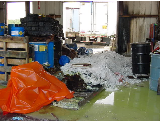
Figure 1: Consolidation Building west side Calcium hypochlorite in center, lithium batteries on left; green water from FD and fire suppression
