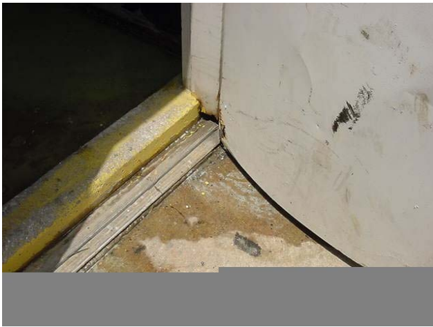
Figure 13: Containment in Consolidation Building leaking
