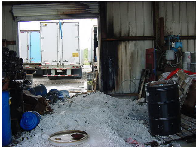
Figure 2: Consolidation Building west side Fire started next to door, up wall
