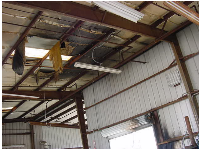
Figure 6: Roof affected by fire
