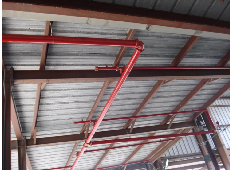
Fig. 2-New fire extinguishing system above loading dock.
