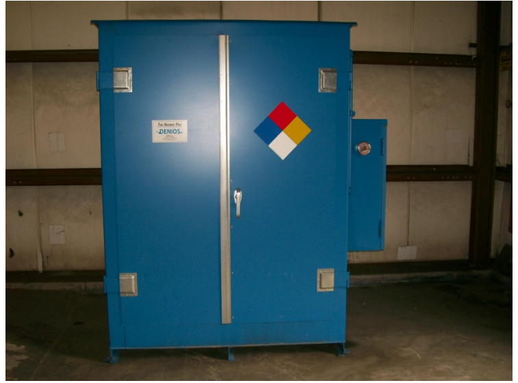
Fig. 8 – Water reactive storage locker within the TSD
