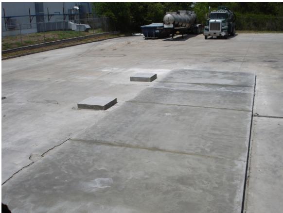
Figure 3-Concrete pad for UO Tank
