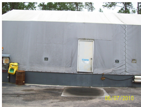
D. Tank Storage
