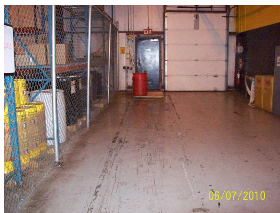
B. Transfer Area
