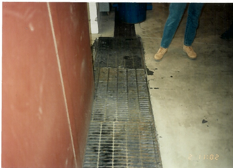
Photo 10b. Trench within the Drummed Flammable Waste Storage Room (SWMU 10). This trench is positioned in front of the sliding door to the Drummed Flammable Waste Storage Room (SWMU 10).
