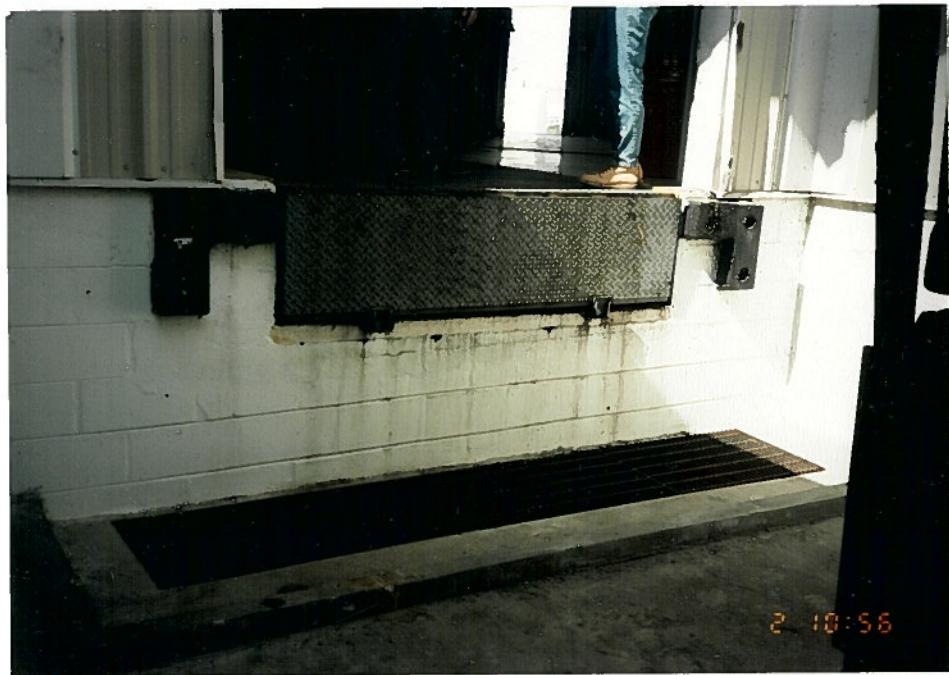
Photo 9b. This sump is located outdoors within one of the Drummed Waste Loading Docks (SWMU 9). The other two loading docks also have sumps positioned in similar layouts.
