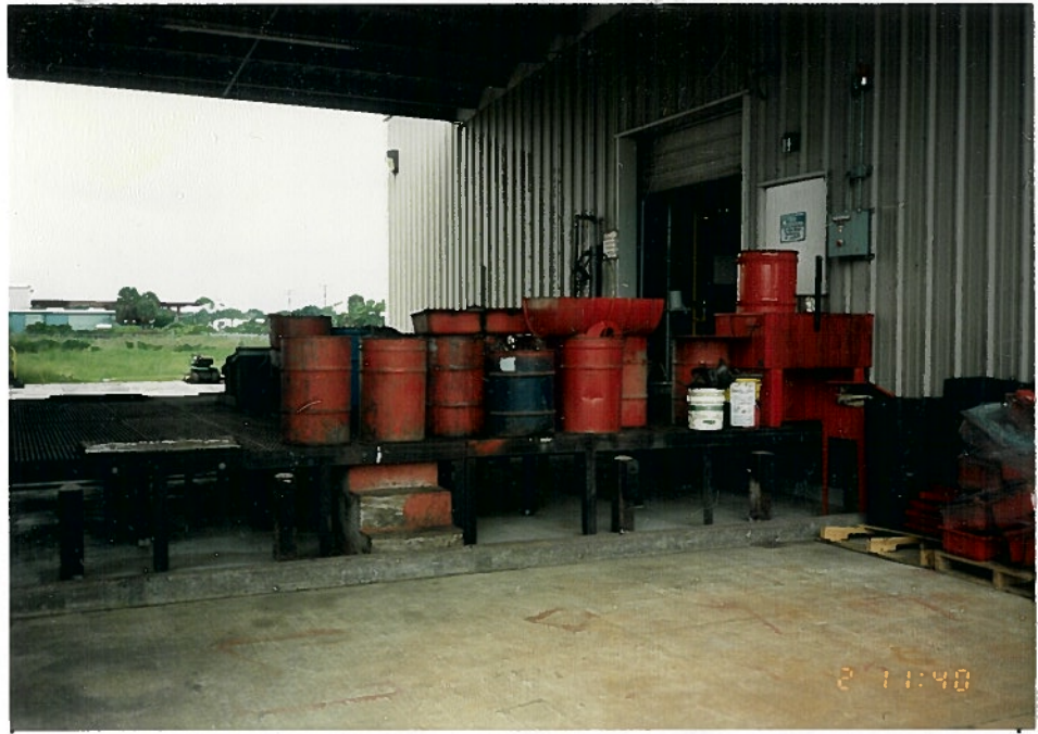
Photo 5a. Overview of the Drum Rinsing Area (SWMU 5). The drum-washing apparatus is the 55-gallon drum that has a halved 55-gallon drum positioned lengthwise over it. This area is located above the Spill Containment Area Below the Fill Shelters (SWMU 4).
