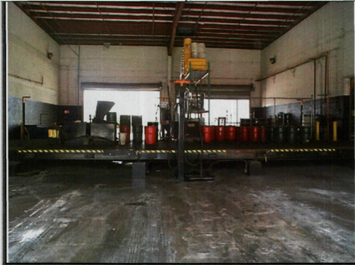
Photograph 1: Return/fill station; view looking northward.
