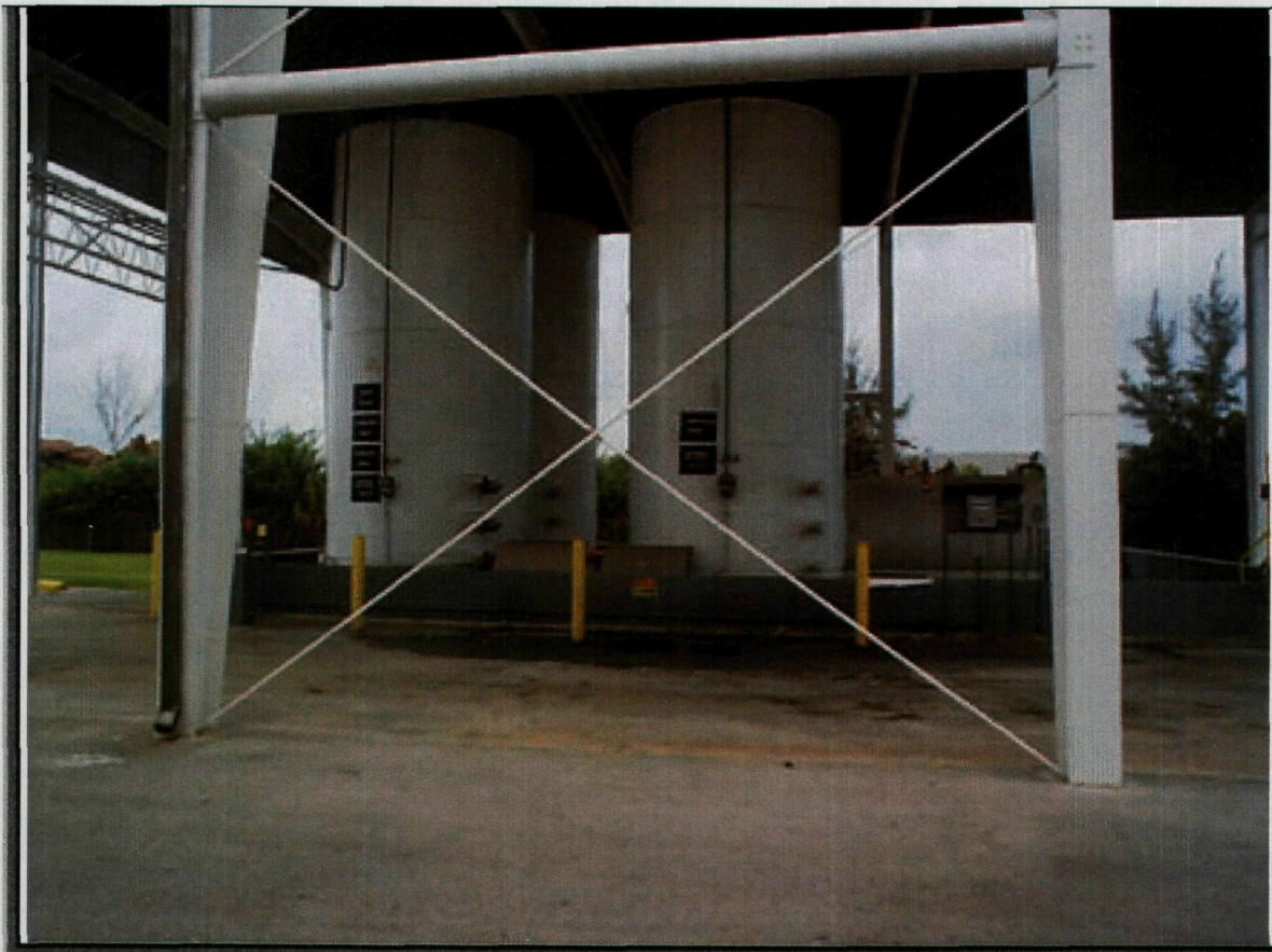
Photograph 6: Tank storage area; view looking northward.
