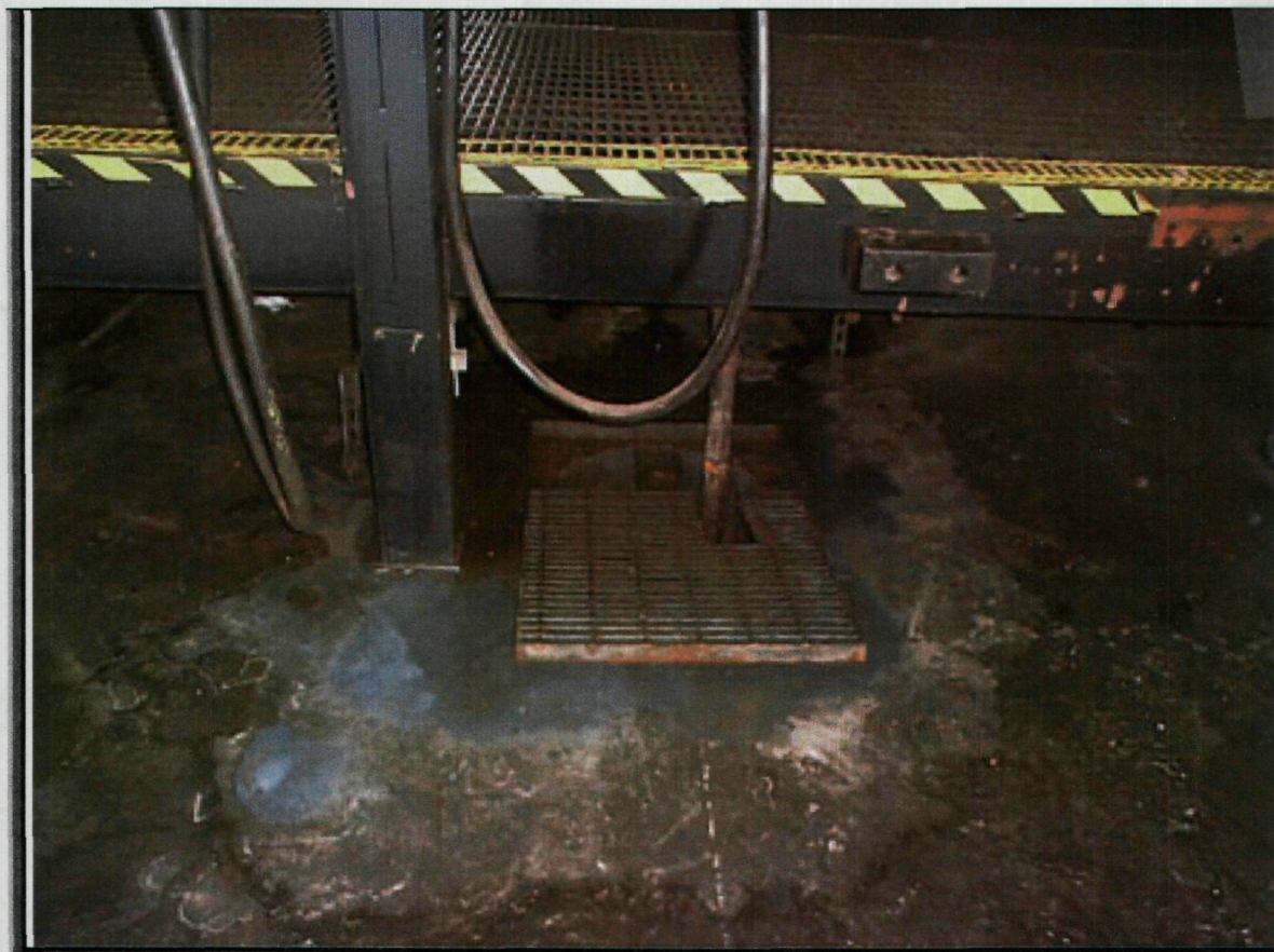
Photograph 2: Containment sump beneath return/fill station; view looking northward beneath the grating.
