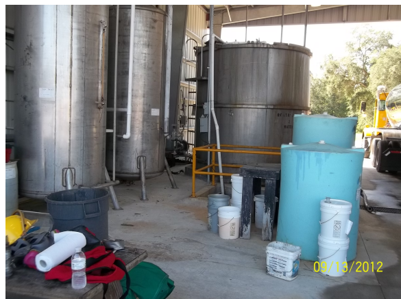
Restricted wastewater tank and leak detection scrubber system
