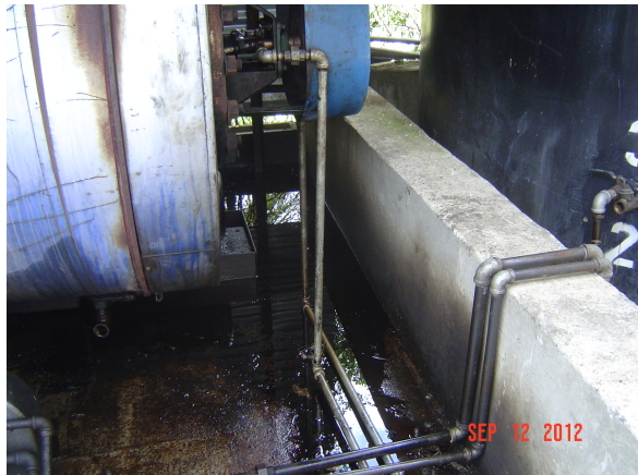
Photo 3 - used oil leak
