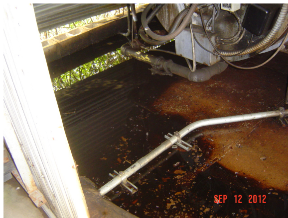
Photo 2 - used oil leak from heater
