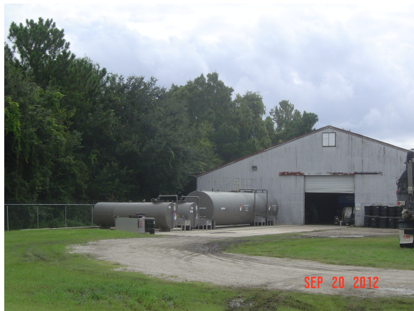
Photo 1 - area for tank expansion
