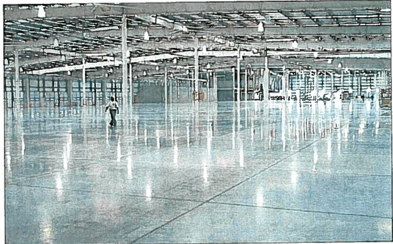
Wal-Mart facility, Guadalajara, Mexico
