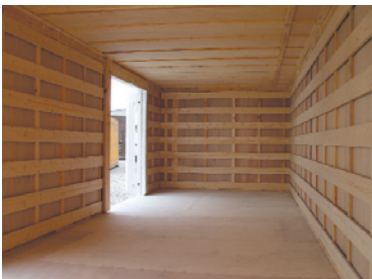
Interior view of 24' x 8' x 8' Type 2 magazine
