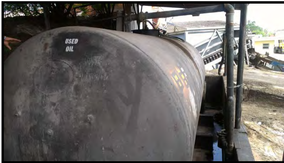
Photograph No. 4 – View of Containment Dike #1b and 5,000-gallon waste oil AST.
