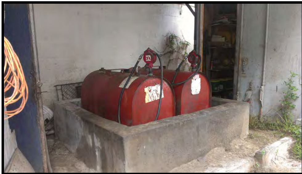
Photograph No. 2 – View of Containment Dike #2 with one (1) 250-gallon motor oil (left, Tank #4) and one (1) hydraulic oil (right, Tank #5) ASTs.
