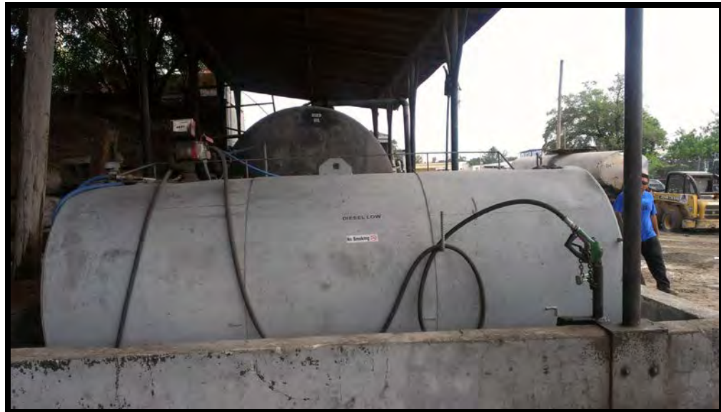
Photograph No. 1 – View of Containment Dikes #1a and #1b with diesel fuel ASTs and waste oil AST.
