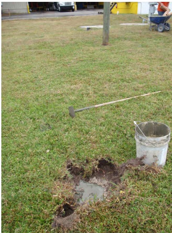
Monitoring Well MW-3 Abandonment Completion
