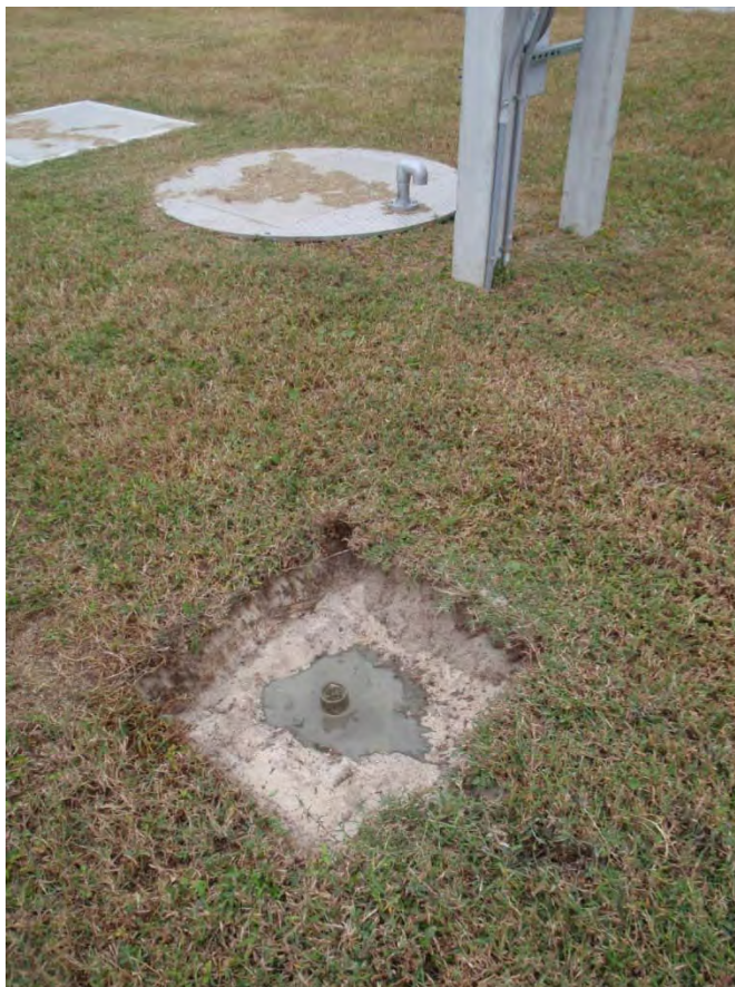
Completed Grouting (Abandonment) of Monitoring Well MW-2 (typical)
