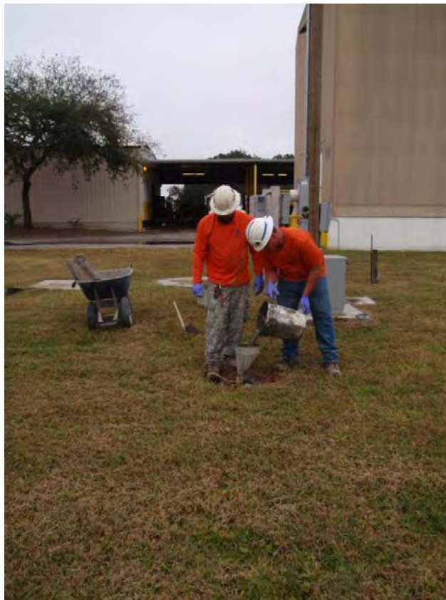
Monitoring Well MW-6D Abandonment
