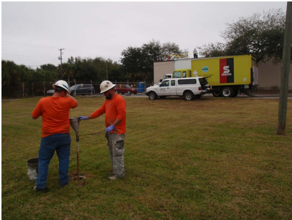
Monitoring Well MW-3 Abandonment
