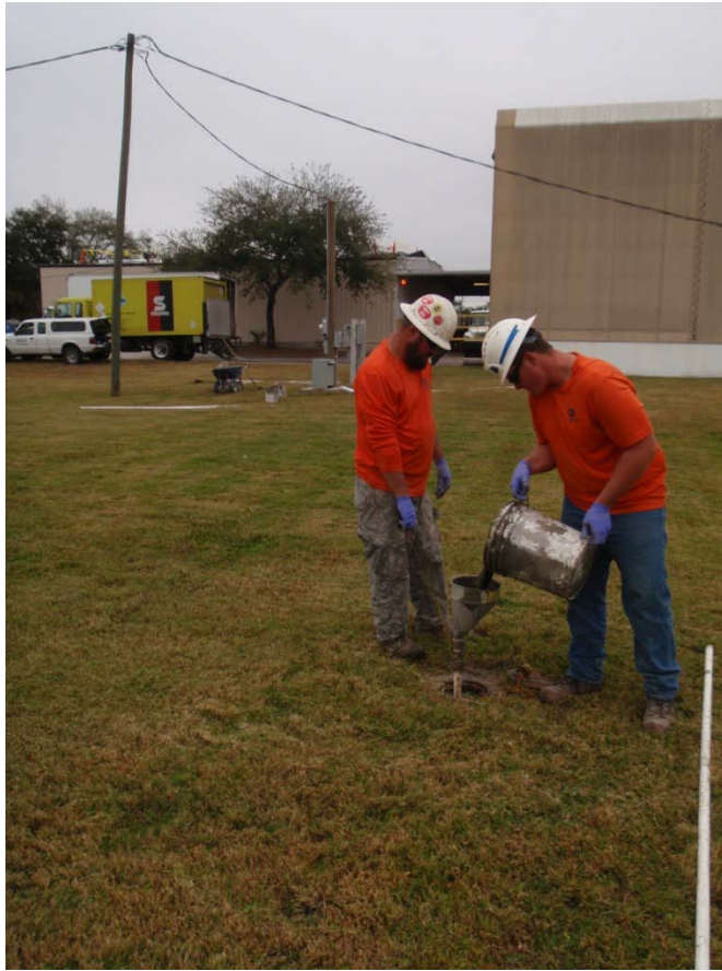
Monitoring Well MW-4 Abandonment
