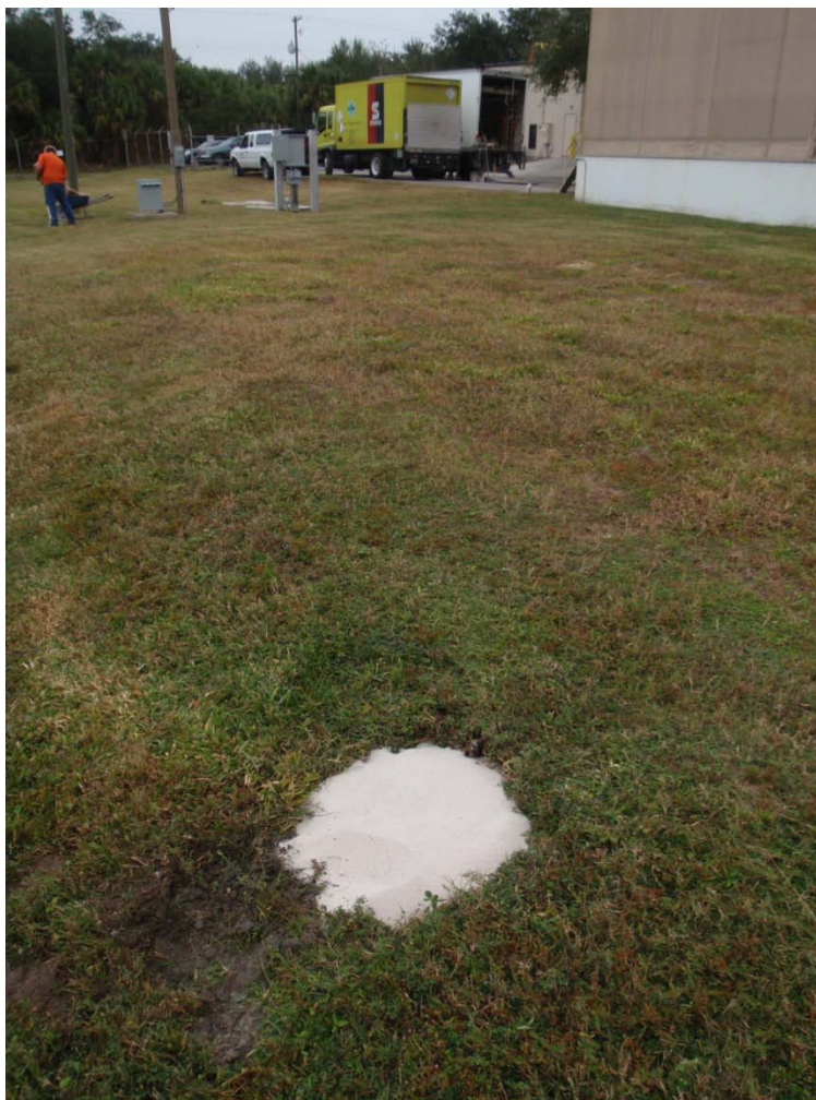
Monitoring Well MW-1 Abandonment Completion (typical)
