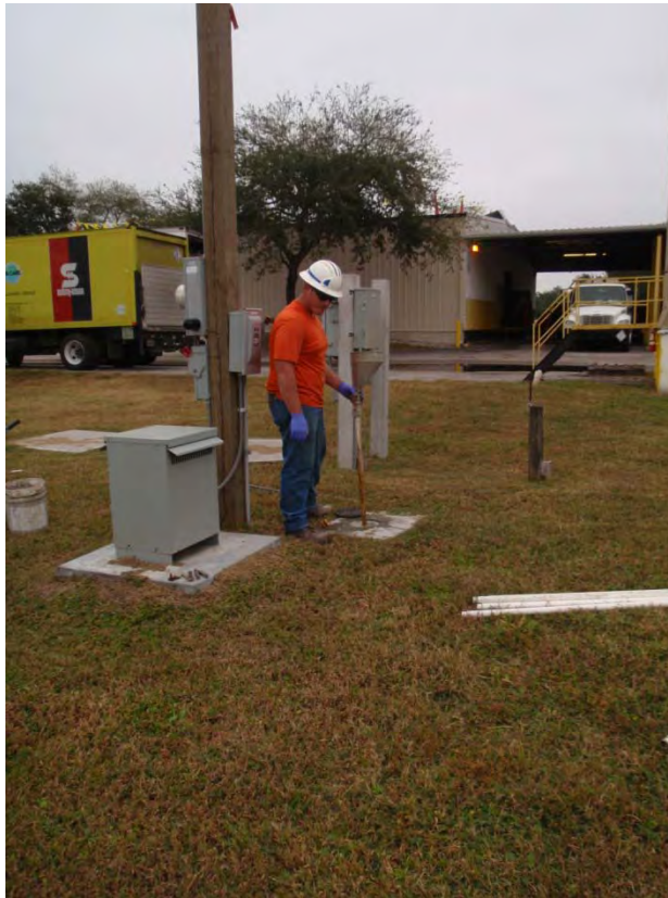
Monitoring Well MW-2 Abandonment
