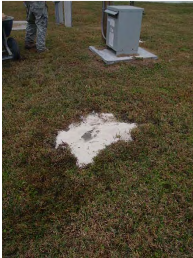
Monitoring Well MW-6D Abandonment Completion
