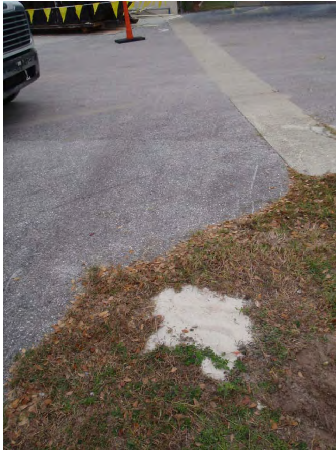
Monitoring Well MW-5 Abandonment Completion
