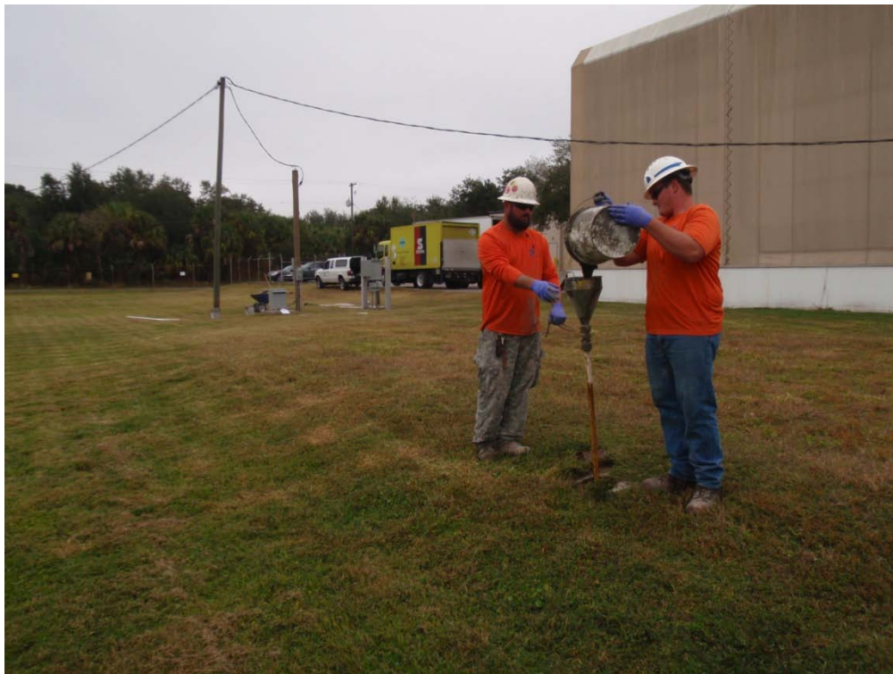
Monitoring Well MW-1 Abandonment
