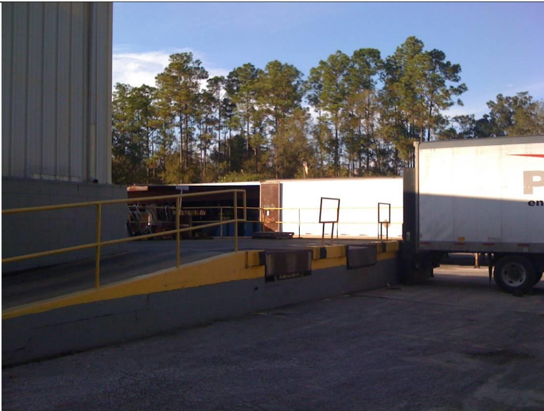
4. East Loading Dock
