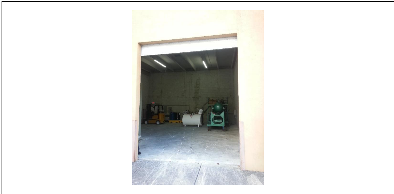
Description: View of Overhang Roll off Door showing AST and LYE-1000 Regeneration System facing South
