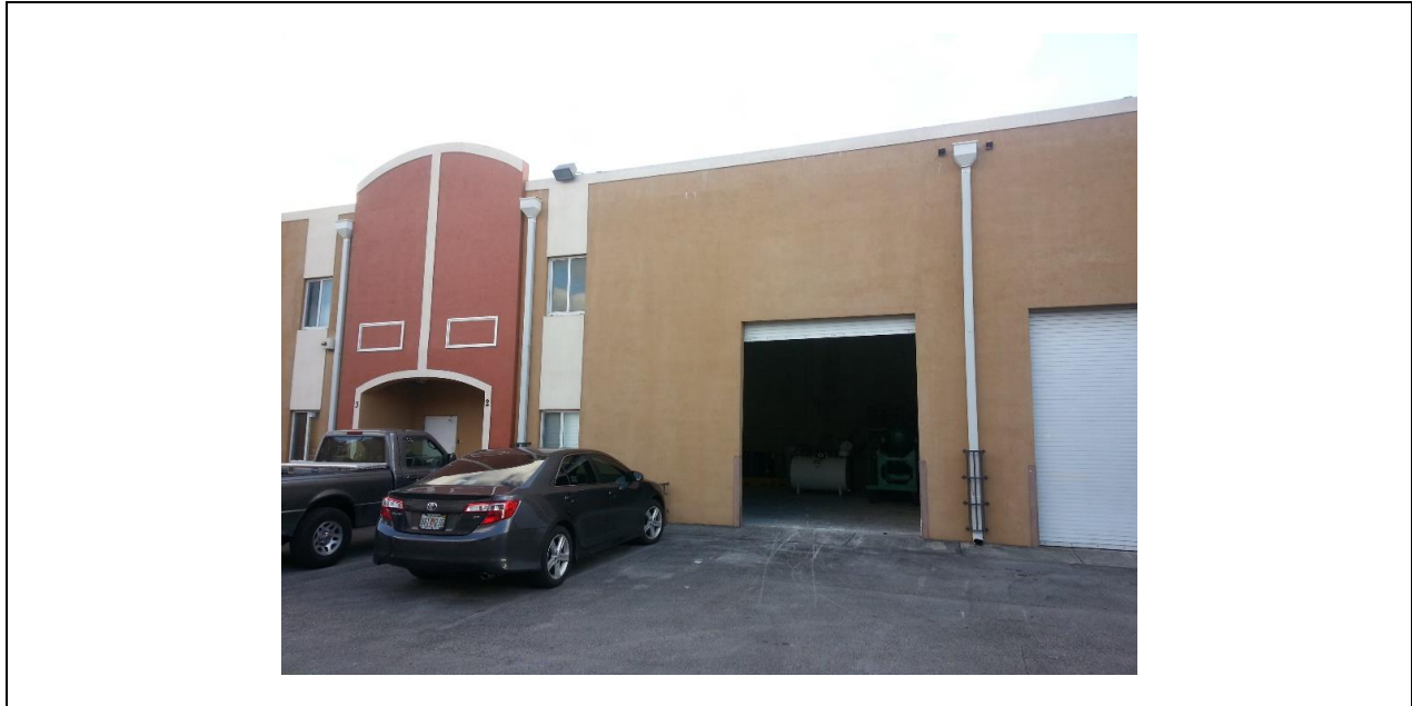
Description: View of the 7855 NW 2 nd Ct Bay 2 Unit showing Overhang Roll off Door facing South
