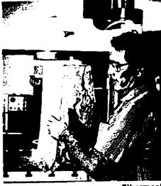
Research engineer removes Fibermesh specimen after test ended. Column was compressed 10% and still remained intact.
