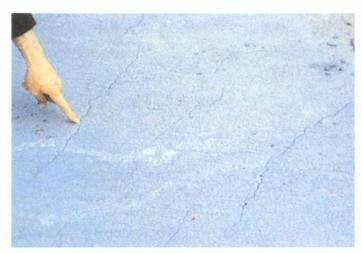
**14.** Typical plastic shrinkage crack. Plastic shrinkage cracks destroy the integrity of the concrete and permit easy access of destructive elements to the reinforcing steel.
