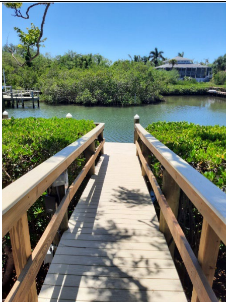
Photo 1: View of the dock facing south.
