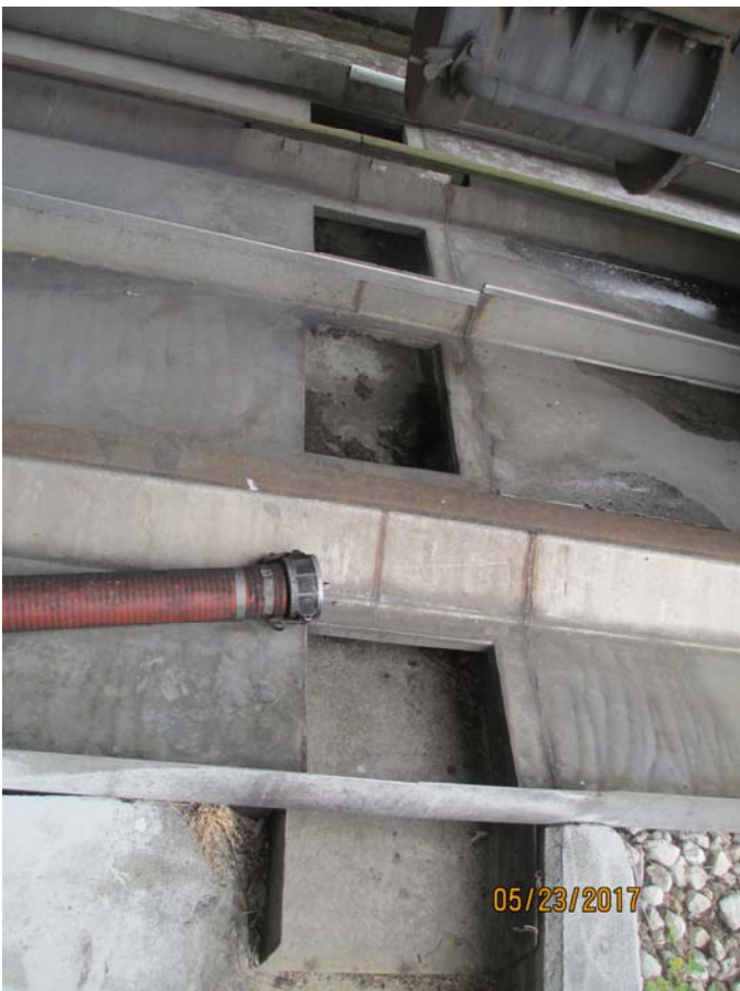
Photo ID # IMG_2475: A track pan is located under the railroad tracks where the rail car is located.
