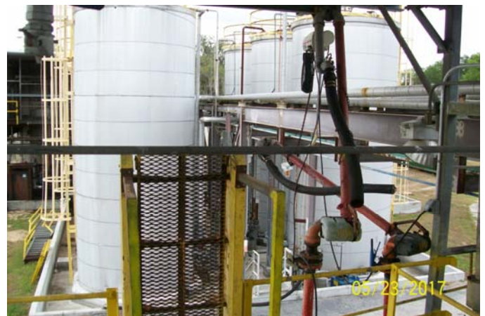
Photo ID # 101_0041: The facility has six 25,000-gallon aboveground storage tanks for the storage of used oil.
