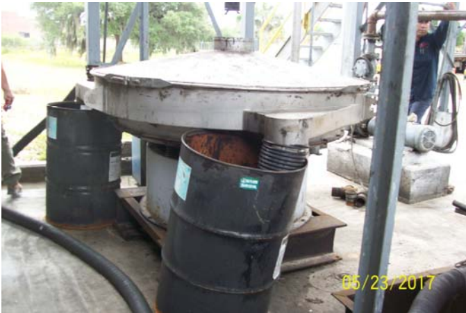
Photo ID # 101_0036: A filter housing located in the loading rack area; the drums collect filtered oil and oily debris.
