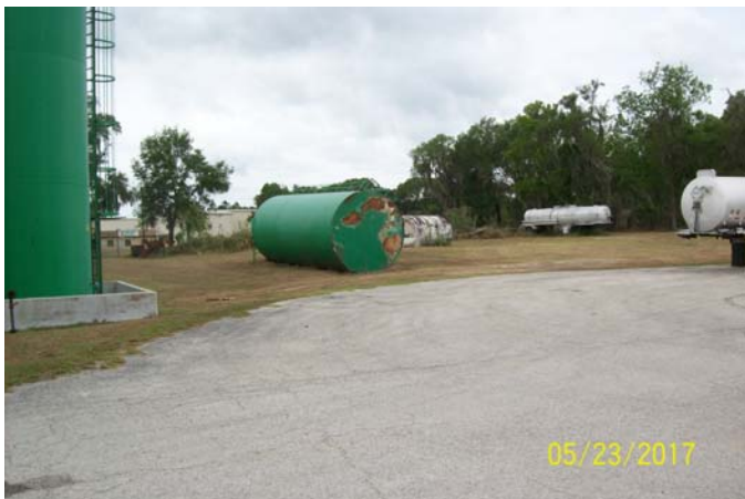
Photo ID # 101_0044: The aboveground green tank installed within secondary containment is empty as are the two storage tanks laying in the yard.
