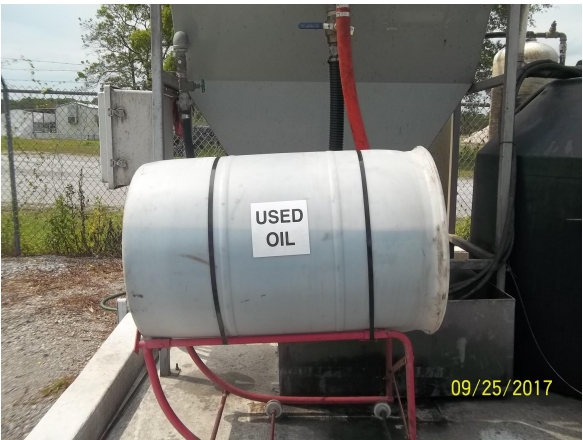
Photo 5 - Labeled Used Oil sludge: water/oil separator
