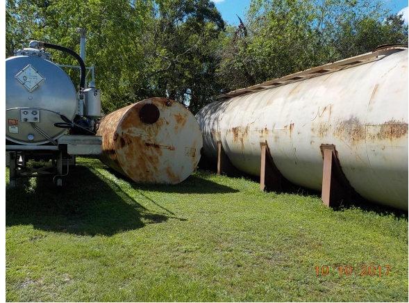
Photo 10, Tanks 1 and 2 of 7 waiting installation
