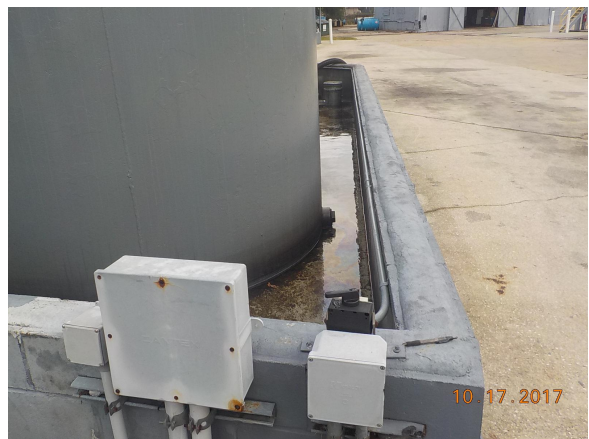
Photo 12 Oily Water Inside Secondary Containment Back
