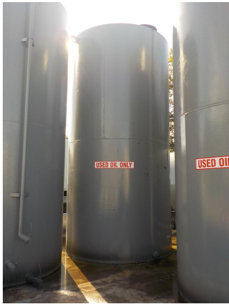
Photo 7 6,000-Gallon Used Oil Tank
