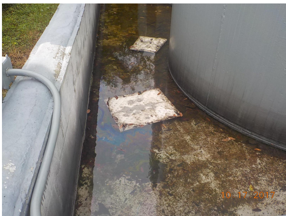
Photo 11 Oily Water Inside Secondary Containment Left Side
