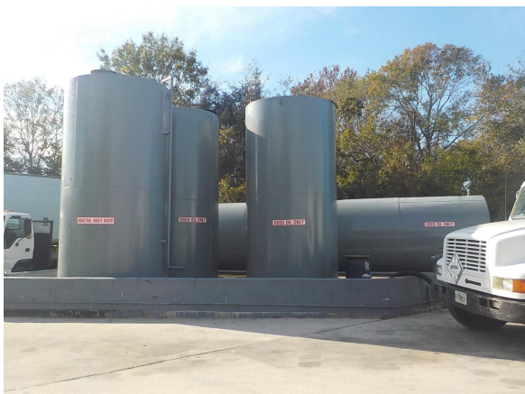
Photo 5 Used Oil and Industrial Waste Water Tanks
