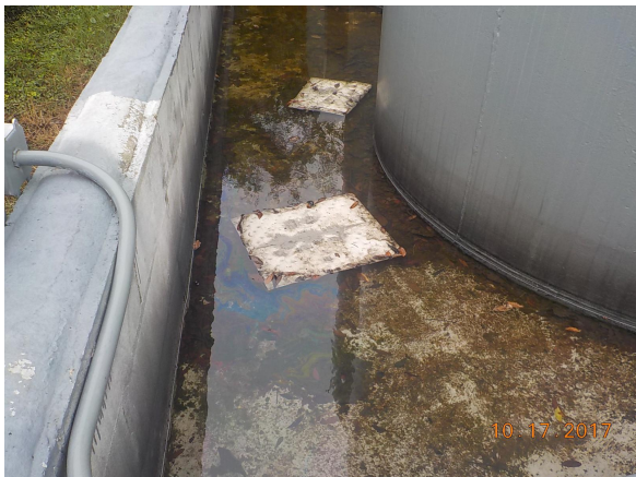
Photo 11 Oily Water Inside Secondary Containment Left Side
