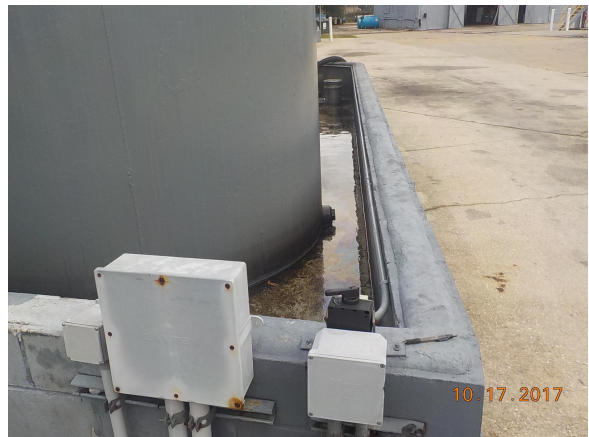
Photo 12 Oily Water Inside Secondary Containment Back
