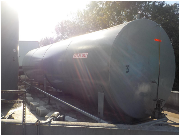
Photo 9 12,000-Gallon Used Oil Tank
