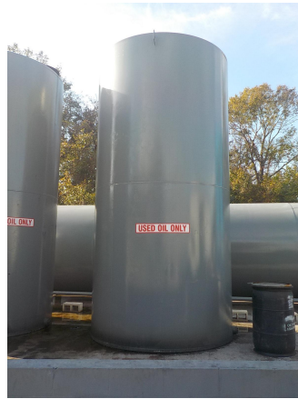
Photo 8 Second 6,000-Gallon Used Oil Tank
