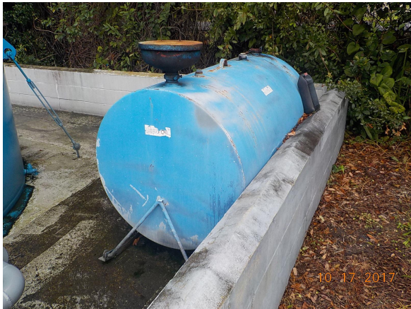
Photo 13 250-Gallon Used Oil Tank
