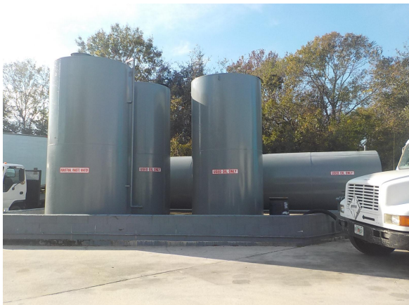
Photo 5 Used Oil and Industrial Waste Water Tanks
