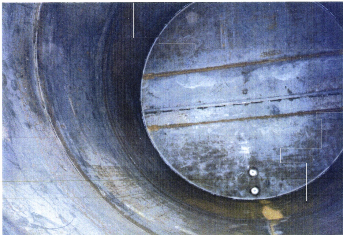
INTERNAL TANK WELDS
