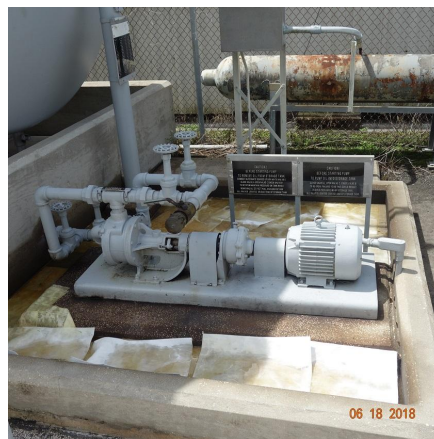
Virgin mineral oil release - pump basin of 25,000 gallon AST
