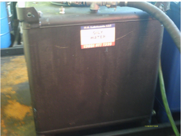
Oily Water Above-Ground Storage Tank (AST) 1
