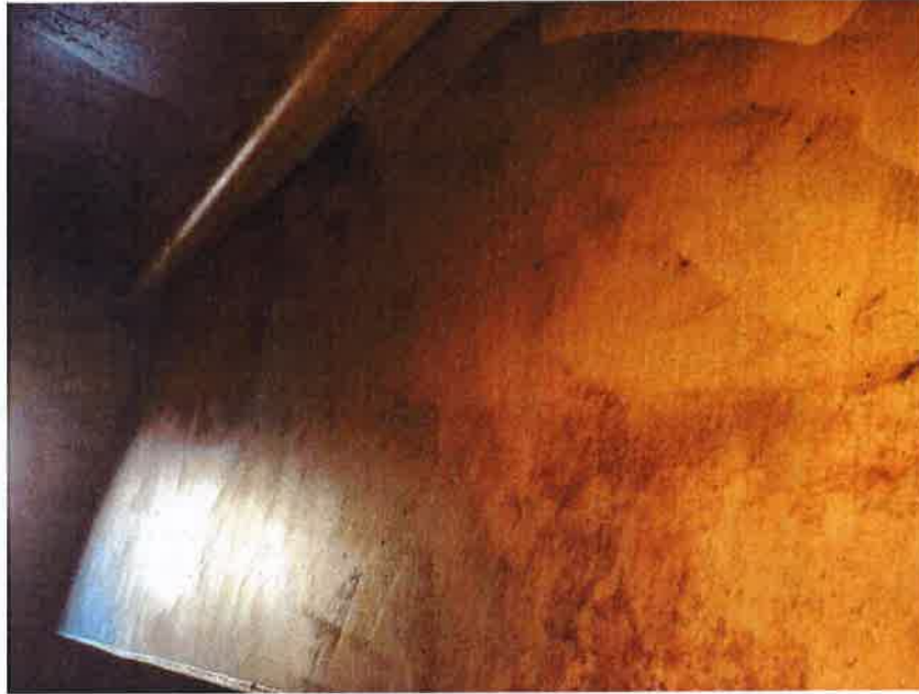
COATING ON SIDE OF WALKWAY RECESS
