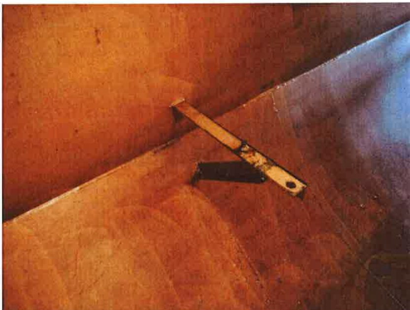
HANGERS FOR REMOVED PIPING AND CLOSE UP OF COATING
