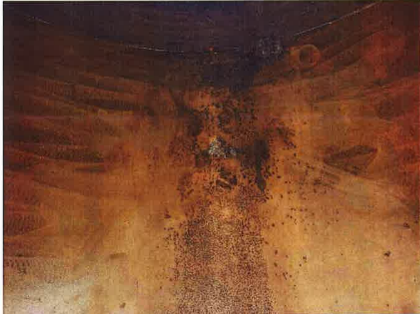
MINOR LOSS OF COATING ON BOTTOM
