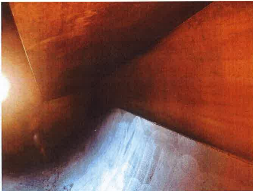
COATING ON BOTTOM OF WALKWAY RECESS
