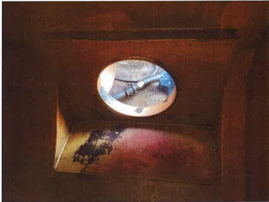
INSTALLATION OF ACCESS HATCH AT FRONT FACE
