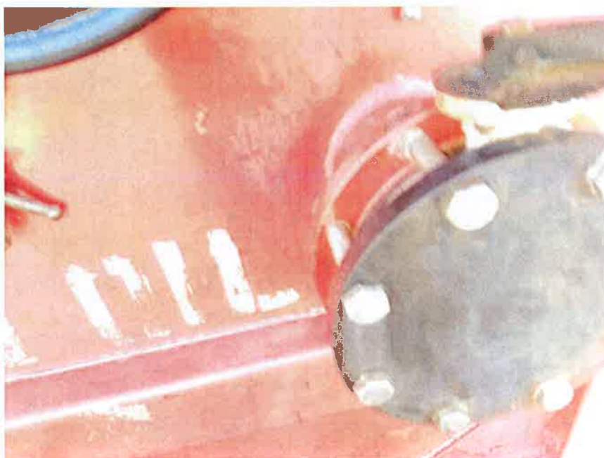
BLANKED FILL / DISCHARGE VALVE
