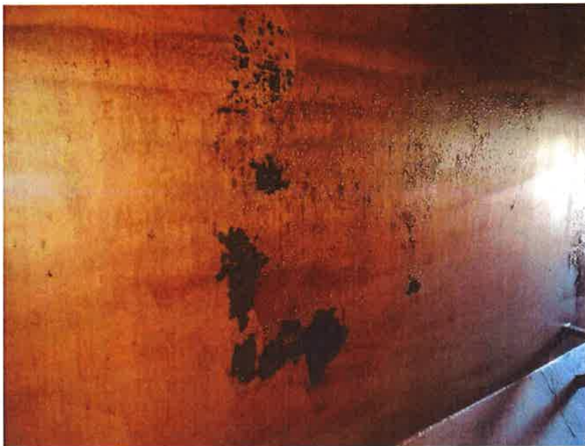
MINOR LOSS OF COATING ON LEFT SIDE
