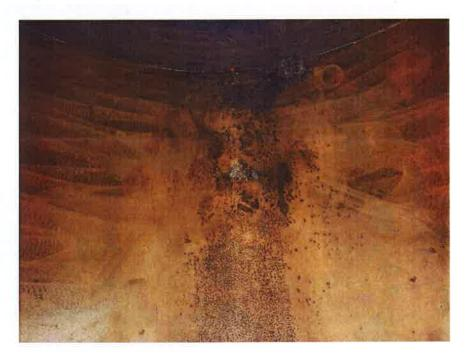
MINOR LOSS OF COATING ON BOTTOM
