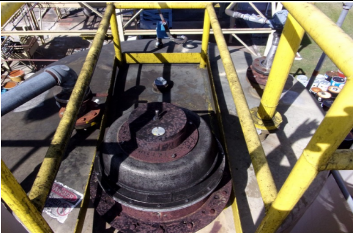
Roof Appurtenances - Condition of hatch(s), manway(s)
