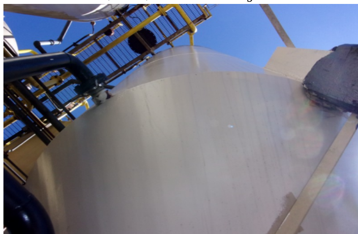
Shell - Coating condition
