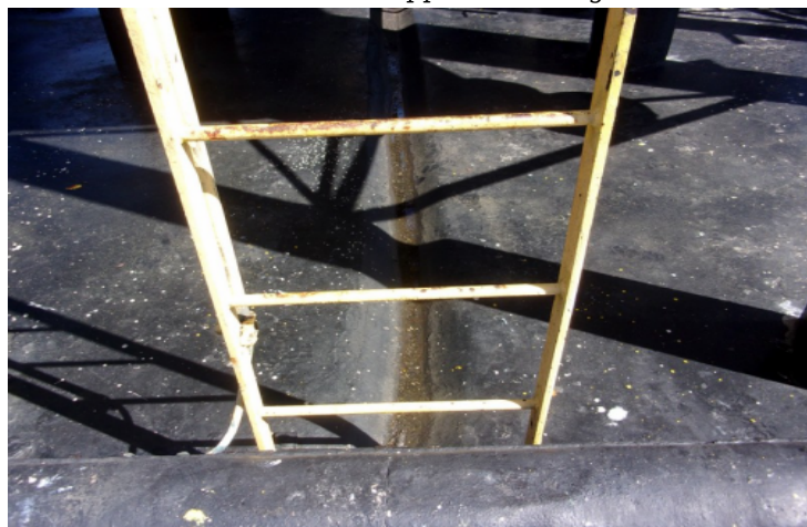
Platforms/Stairs/Ladders - Coating condition
