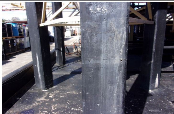
Foundation Support - Coating
