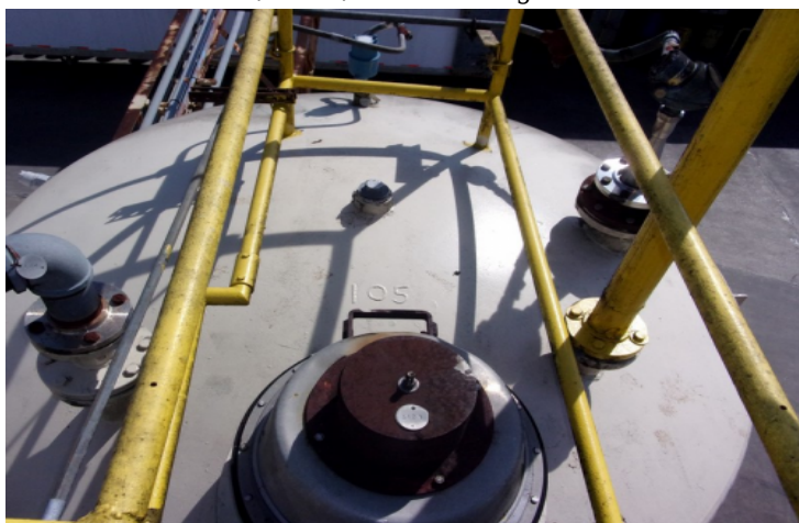
Roof Appurtenances - Condition of hatch(s), manway(s)
