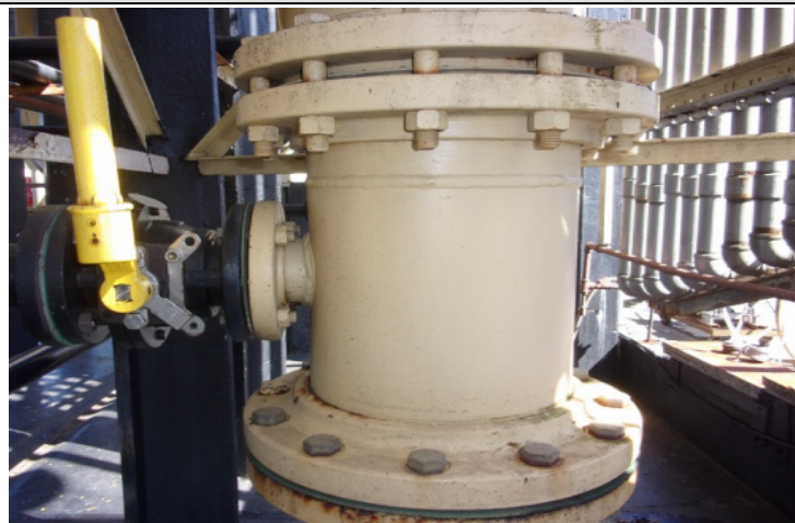
Manways / Nozzles - Bolting condition
