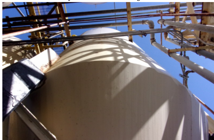
Shell - Coating condition
