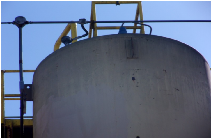
Shell - Coating condition
