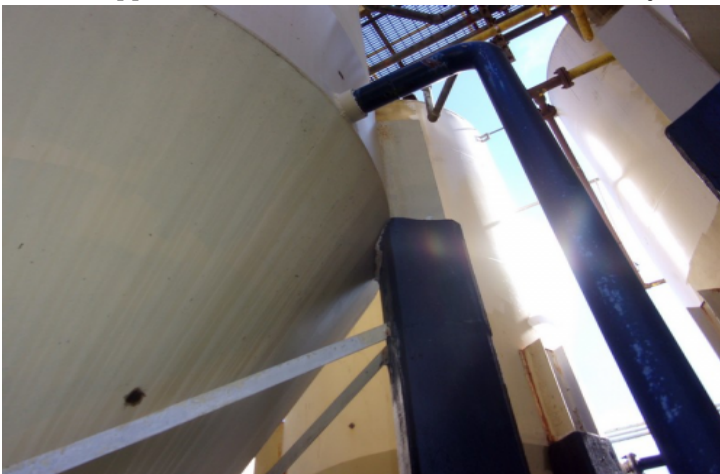
Shell - Corrosion / Pitting
