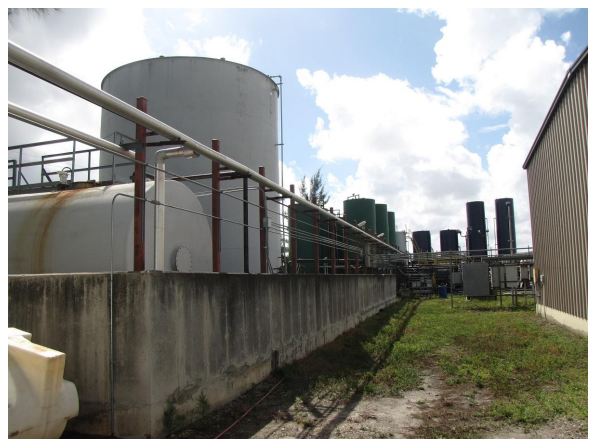
North Tank Farm
