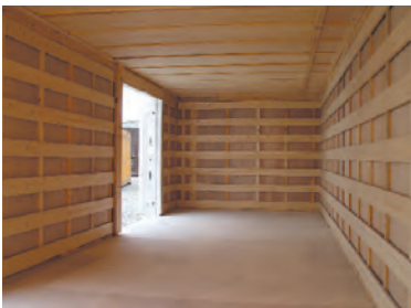
Interior view of 24' x 8' x 8' Type 2 magazine
