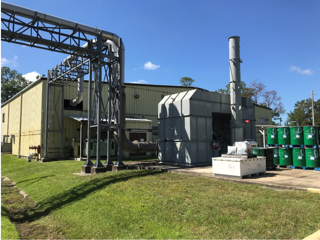
Photo 5. Regenerative Thermal Oxidizer (RTO) (09/2019)
