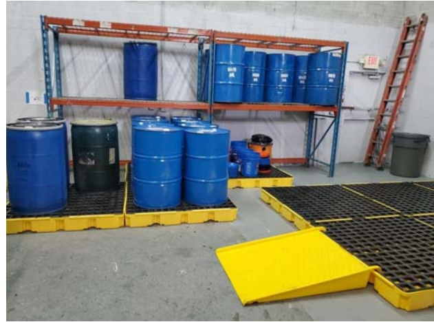
UO drums with secondary containment
