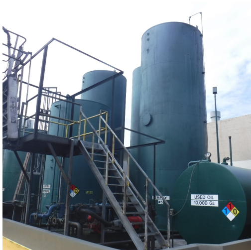
Tank farm located in secondary containment
