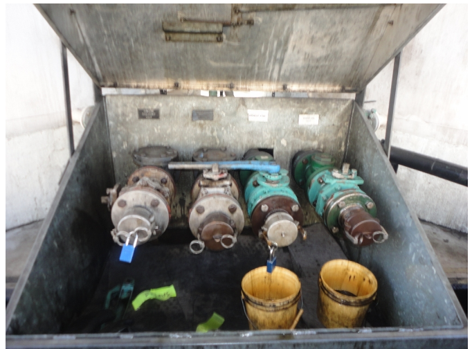
4. Tank spill bucket and fill ports
