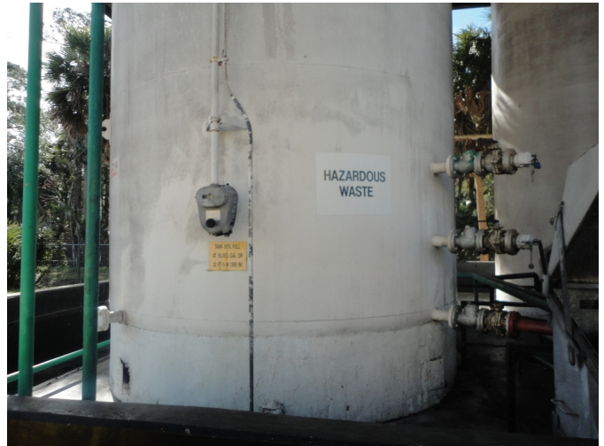
4. Tank spill bucket and fill ports
