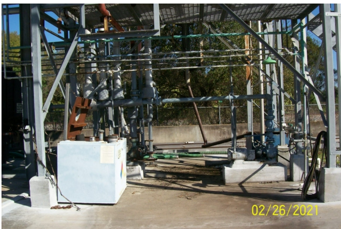
Overhead used oil loading rack
