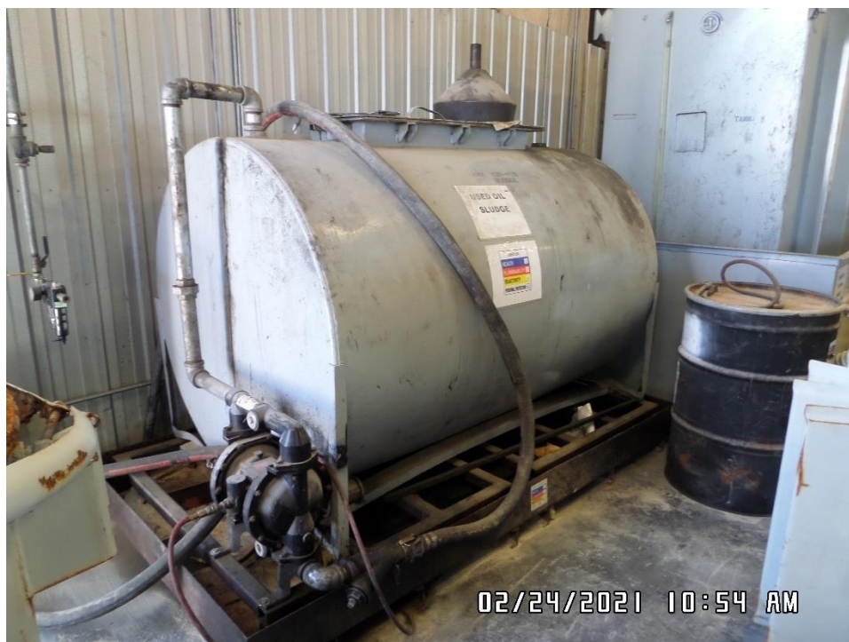
Figure 2 - Used Oil AST with secondary containment
