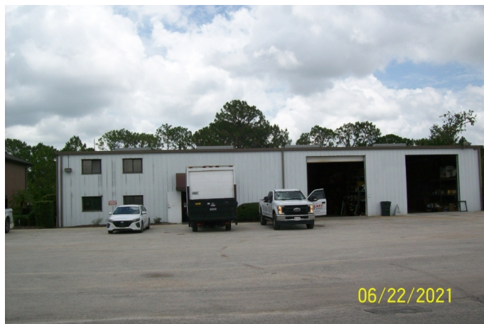
Overview of Warehouse #1
