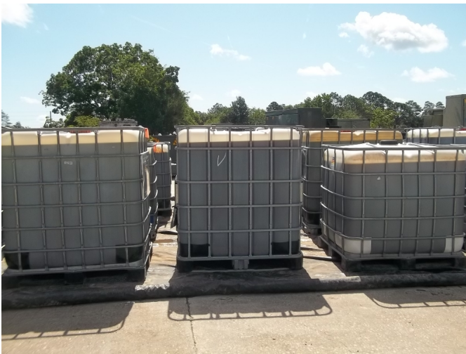
Photo 3: Temporary Secondary Containment for IBC Tote Area
