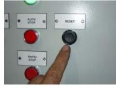
Press Auto Start and the system will now run through sequential start-up, with the exception of the Universal Rumbler, conveyor and crusher. When the Auto Start is pressed the siren and light on top of the cabinet sounds for 3-5 seconds to warn people the system is starting.
