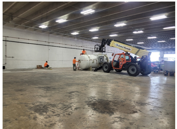
Biohazard waste processor being installed at HES
