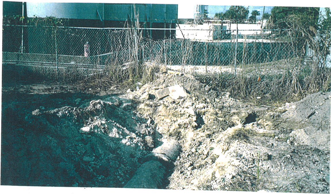
PLATE I: North Test Pit excavation facing northwest. Concrete drainpipe uncovered in foreground. Permafrix aboveground tank farm in background.
