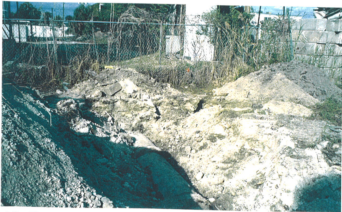
PLATE II: North Test Pit excavation facing north. Concrete drainpipe terminates at chain link fence (property boundary). Permafrix former IRA excavation area in background.
