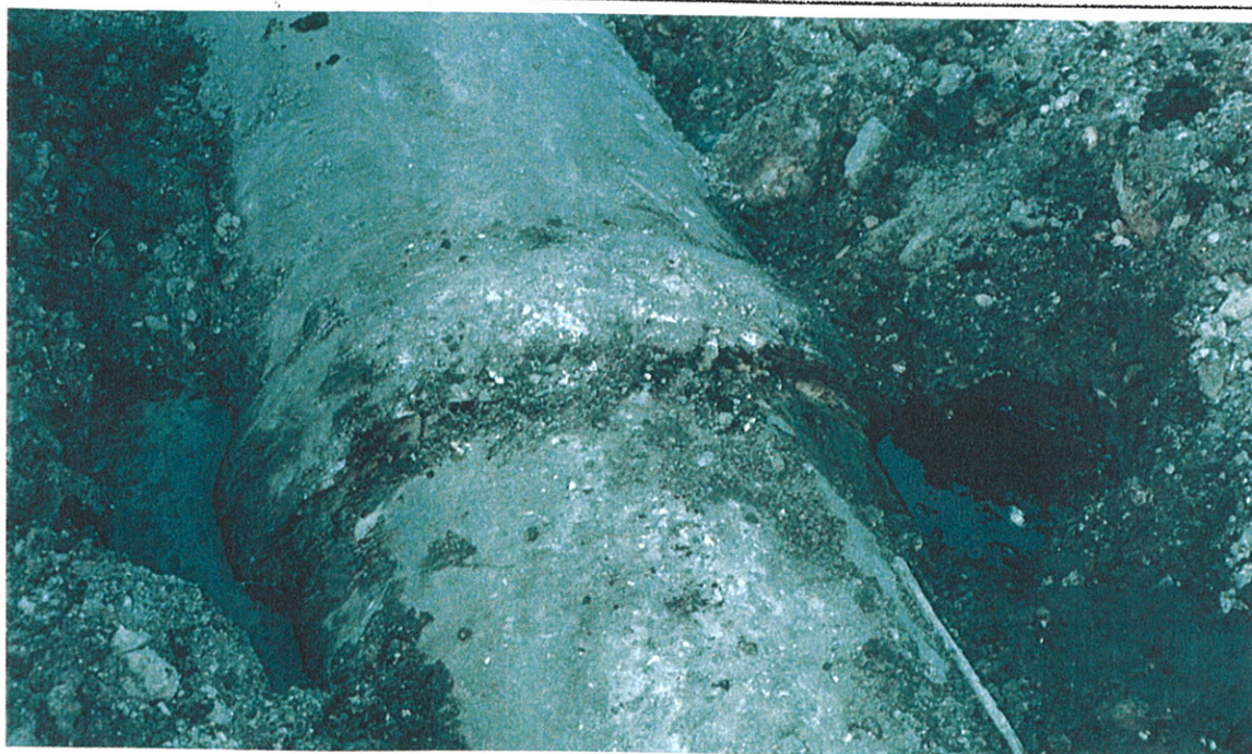
PLATE IV: North Test Pit excavation close up of concrete drainpipe. Note corrosion of pipe coupling allowing seepage of waste petroleum products.
