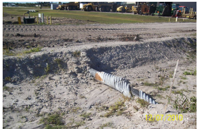
Exposed pipe inside culvert.
