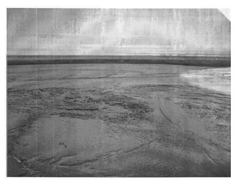
Figure 4 –Approximately 6 to 8 inches of sludge covered the inner tank floor prior to cleaning.
