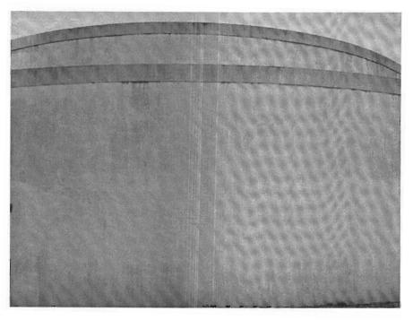
Figure 11 – Minor superficial covercoat cracking was noted on the exterior wall of the secondary containment tank.
