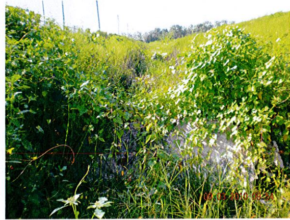
Rock check dam, foreground and mid photo
