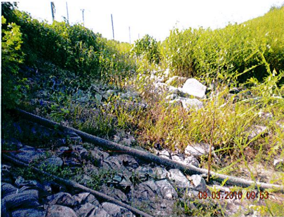
Current condition, vegetation re-established
