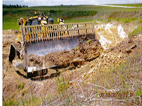
Dozer repairing slope
