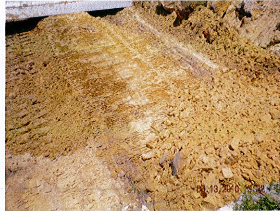
Soils replaced in 12" lifts
