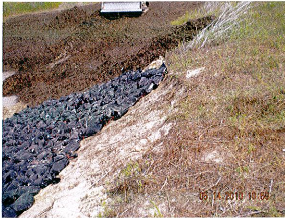
Mulch placed to enhance stabilization
