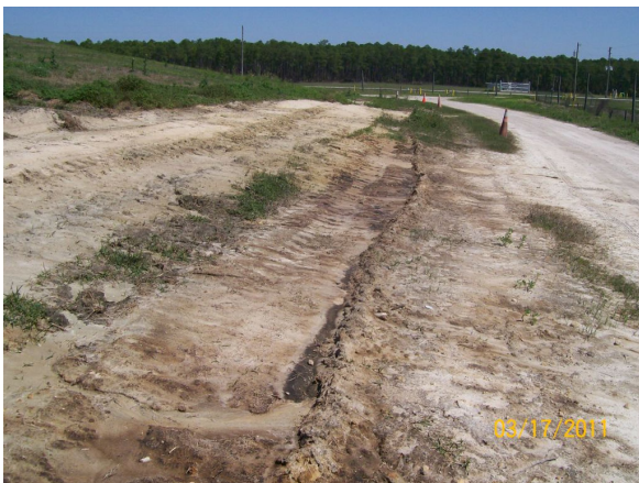
seepage @ recent hog damage repair
