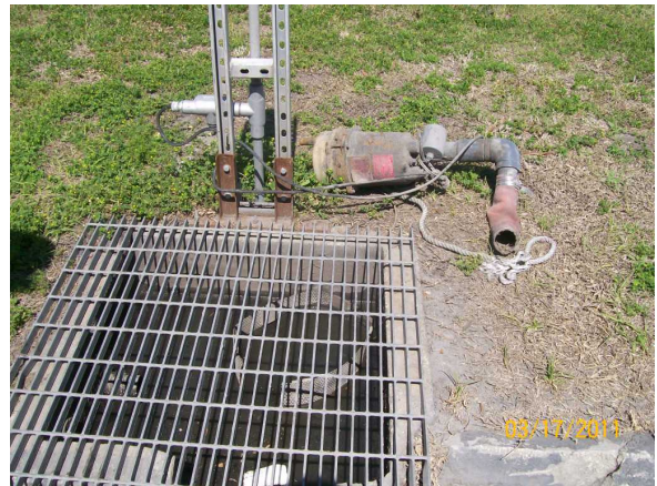
ash bldg drive-way sump pump
