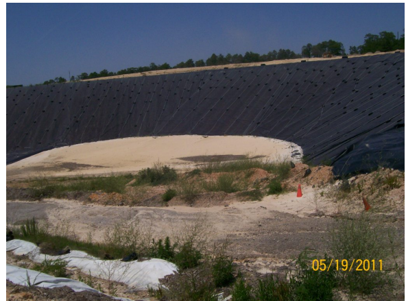
Phase III drainage sand - E side
