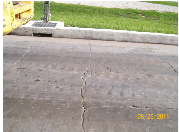
new ash building curbing
