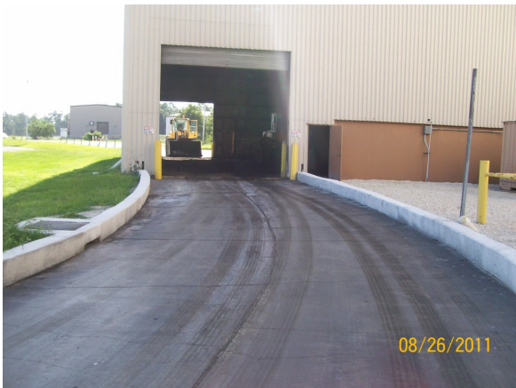
new ash building curbing
