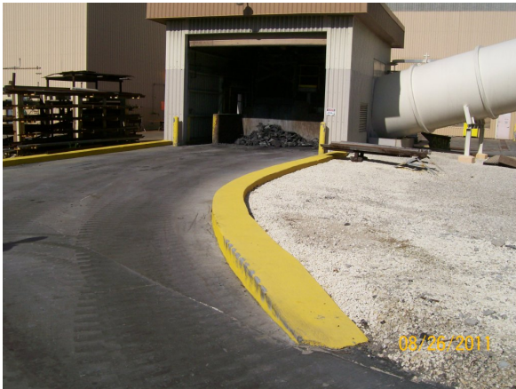
grizzley pavement replacement
