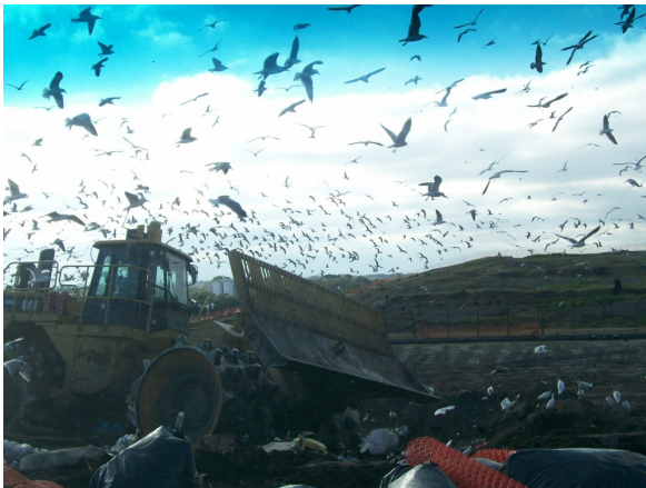
Compactor at working face
