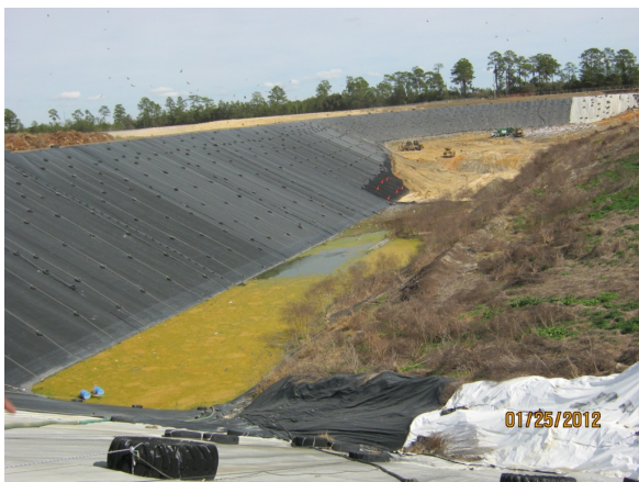
Ponding on rain cover in Phase 3
